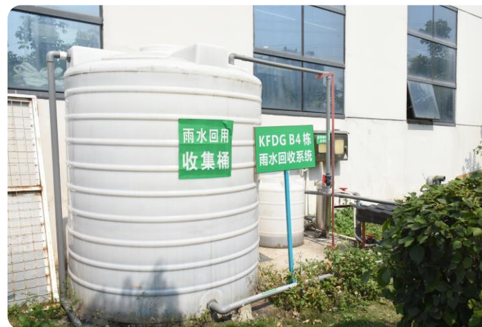
Kaifa Dongguan Rainwater Recycling and Utilization System
